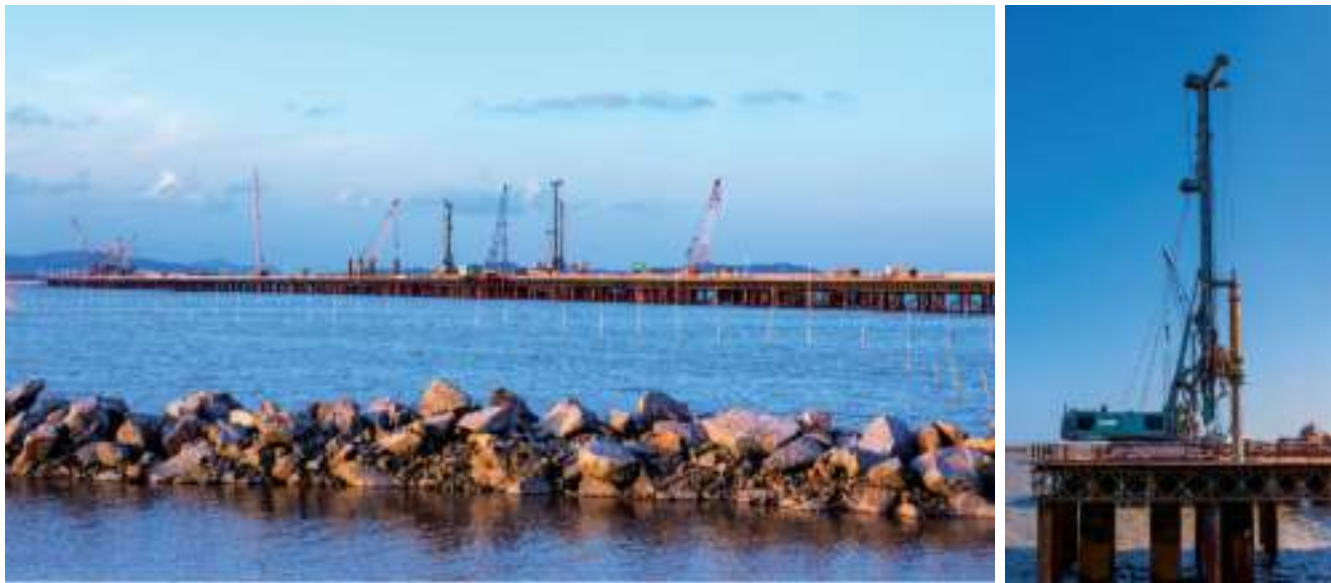
This is Feiyun river bridge construction in Wenzhou. In this project, the construction aperture is 2.2 meters and the depth is about 98 meters which is about 90 meters below the surface. Under the bottom of the sea surface is within 0 ~ 60 meters for silt layer, muddy clay layer, as well as 60 meters for gravel layer. Single-hole drilling a hole is about 7 hours.
