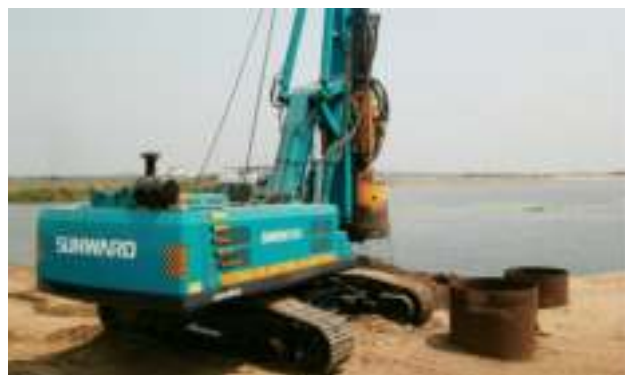
Godavari Bridge - India
