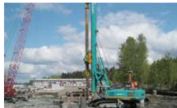
Construction job site - USA
