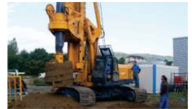
CFA Drilling - France
