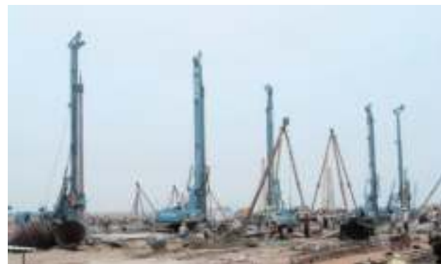
Construction job site - The Ganga River, India
