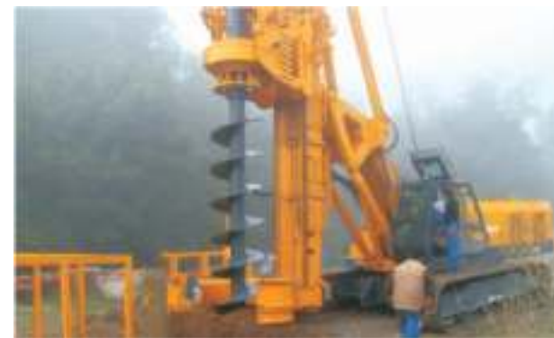
CFA Drilling - Switzerland
