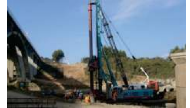
Salerno construction site, Italy
