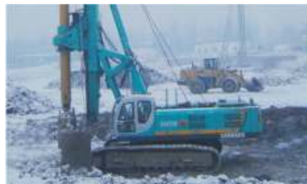
Construction site at -30 - Moscow, Russia
