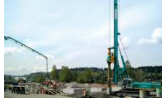
Widening of Azzno Highway in Italy
