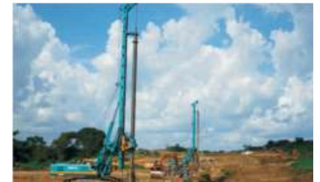
Construction of Tinaco-Anaco Railway - Venezuela
