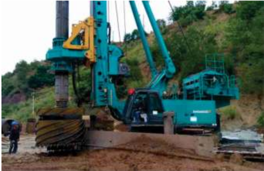
SWDM600W Yunnan high-speed cross Red River grand bridge construction, bearing a complex geological condition with backfill, boulders, gravel layers and other strata. The construction adopted the technology of vibrating hammer retaining cylinder and mud protection wall. The pile diameter is 2.5m, the drilling depth is 72m, and the drilling time is 39 hours for each pile
