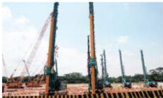
Construction of Metro - Singapore
