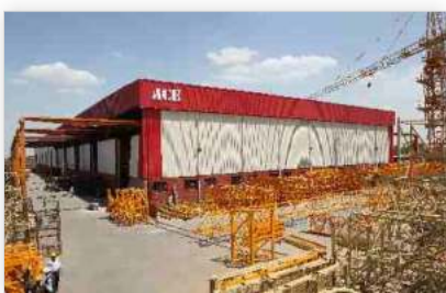
Tower Crane Plant
